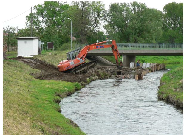
Construction works at Kleinraschuetz begin
