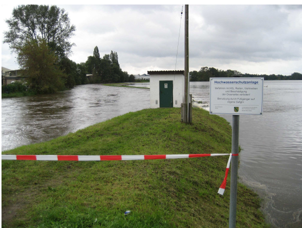
Flooded dike at Kleinraschuetz during the flood in 2010
