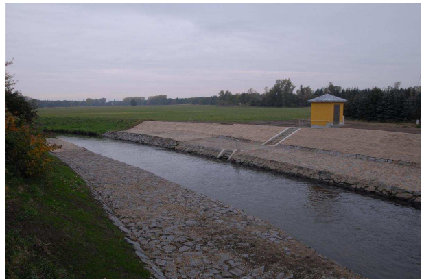
The station at Kleinraschuetz after the installation of the Hybrid system
