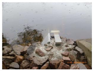
Rebuilt carrier of the lower measurement path with deflector
