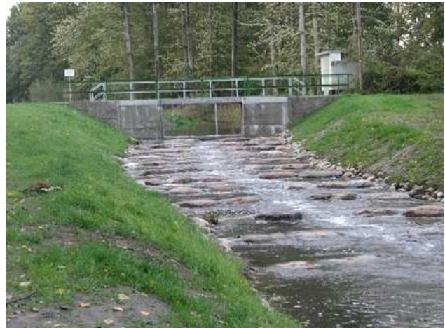
Rock ramp at the Rothentor after completion (Picture: StAUN Schwerin)
